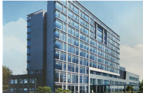
Aerial view of the MND Outplacement Training Institute (construction underway in Wirye New Town)
