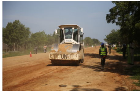
Road repair work
