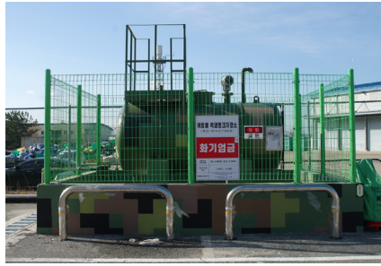
Soil Contamination Prevention System (fuel tank containment dike)
